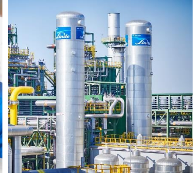
Customised Gas Processing Plants
